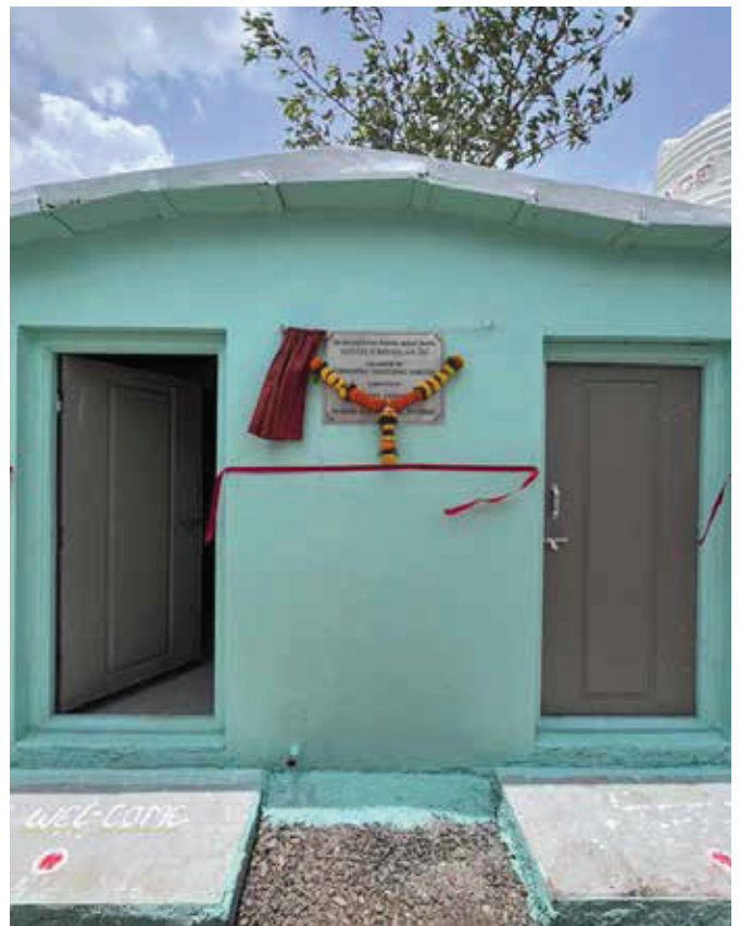
Construction of Toilet, Rajwada School
